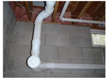
Vent Piping Material The vent material, as it passes through the roof, is plastic.
