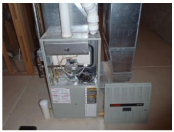
OPERATION OF UNIT: Unit was operating at 90.1% efficiency based on combustion analysis.
